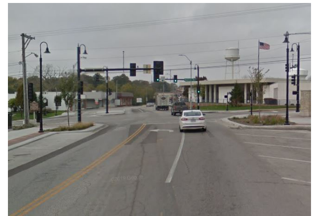
Pavement Marking Project
